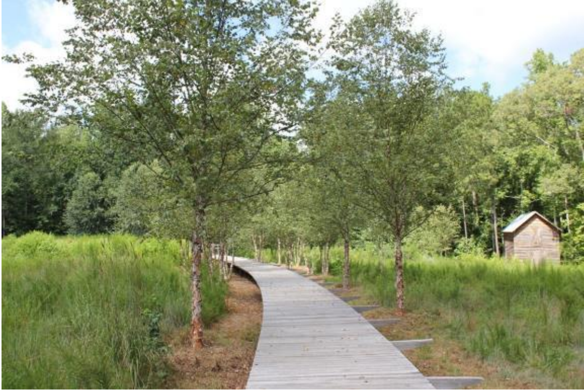
Figure 4.44 Natural Wastewater Treatment Plant
