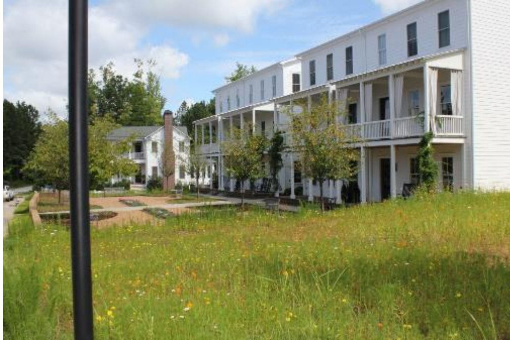
Figure 4.25 Crossroads Townhomes and Courtyard
